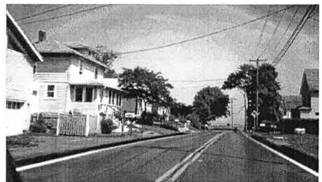
Figure 60 - Simulation illustrating the visual effect of pavement marking variation at the fog line and darkening shoulders to improve awareness of hazard warning signs.
