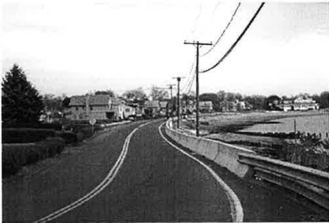
Figure 56 - existing Jersey barrier at Limewood Beach.
