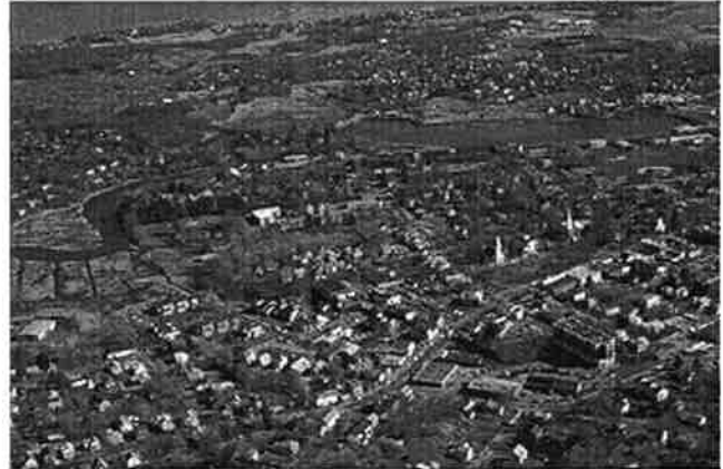
Figure 7 - Aerial view of Branford Center with the Branford River in the background.
